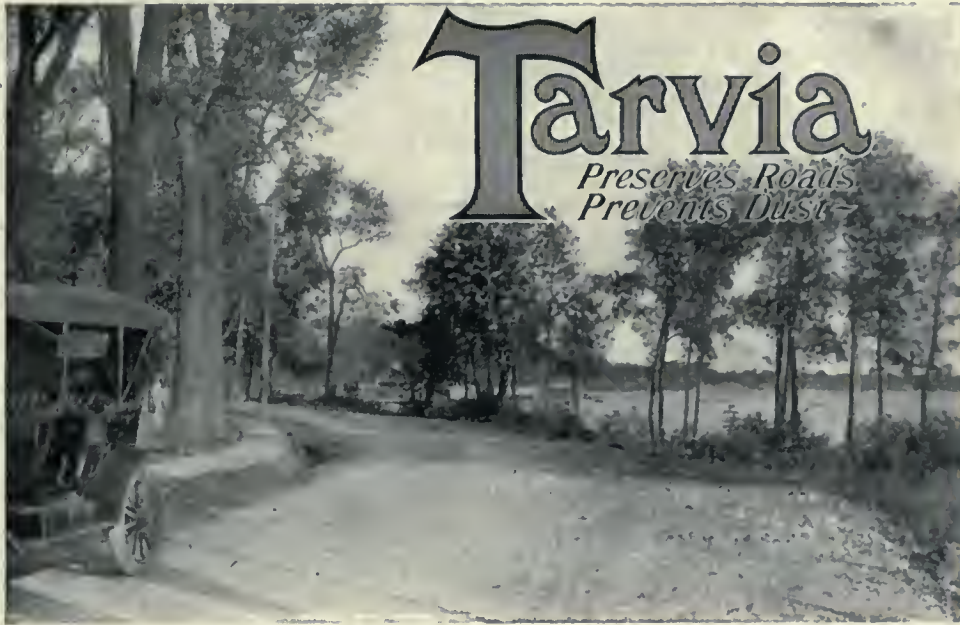
Pointe Claire Road, Quebec. Tarvia Filled Macadam.
